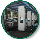
EV Charging Station
